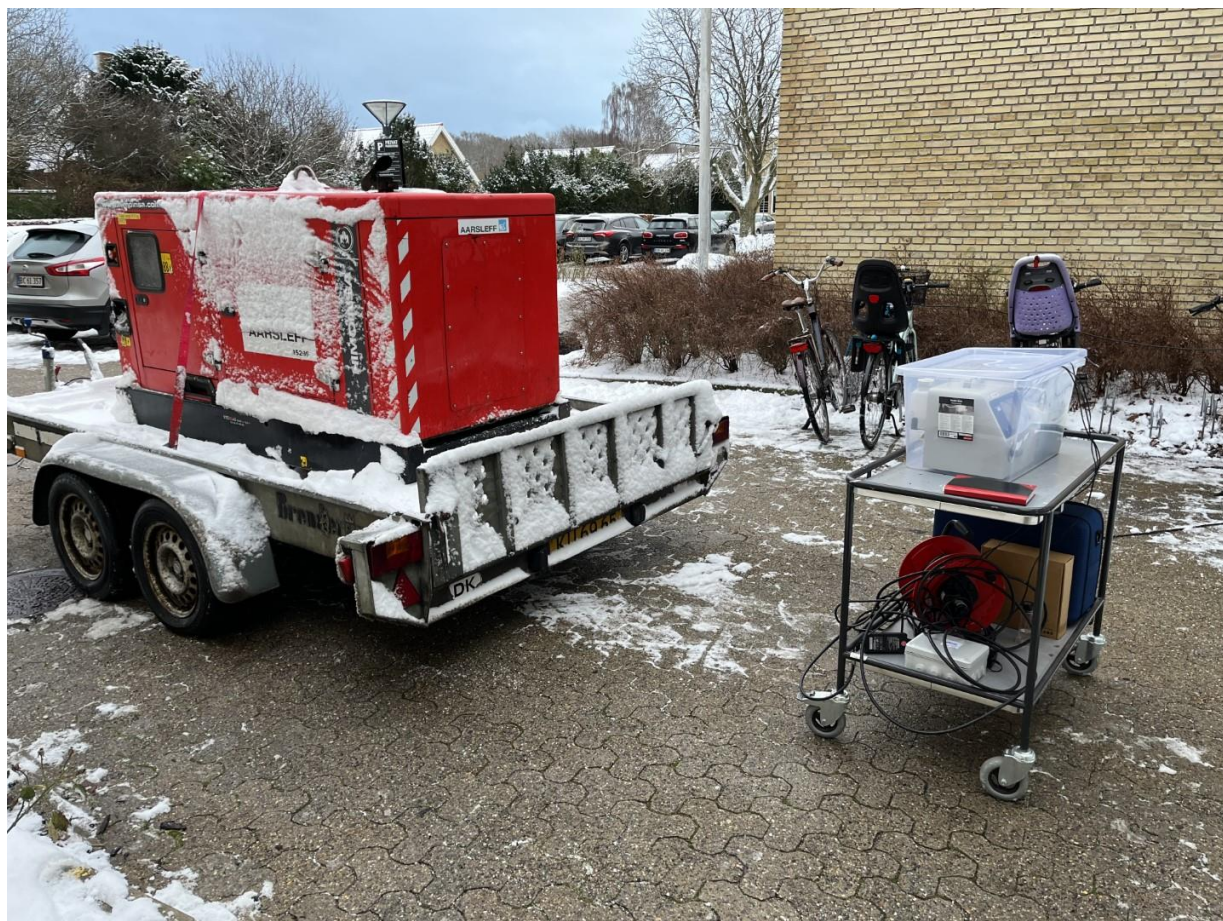
Figure 6. Measurement position 2, 190 cm from the diesel generator.
