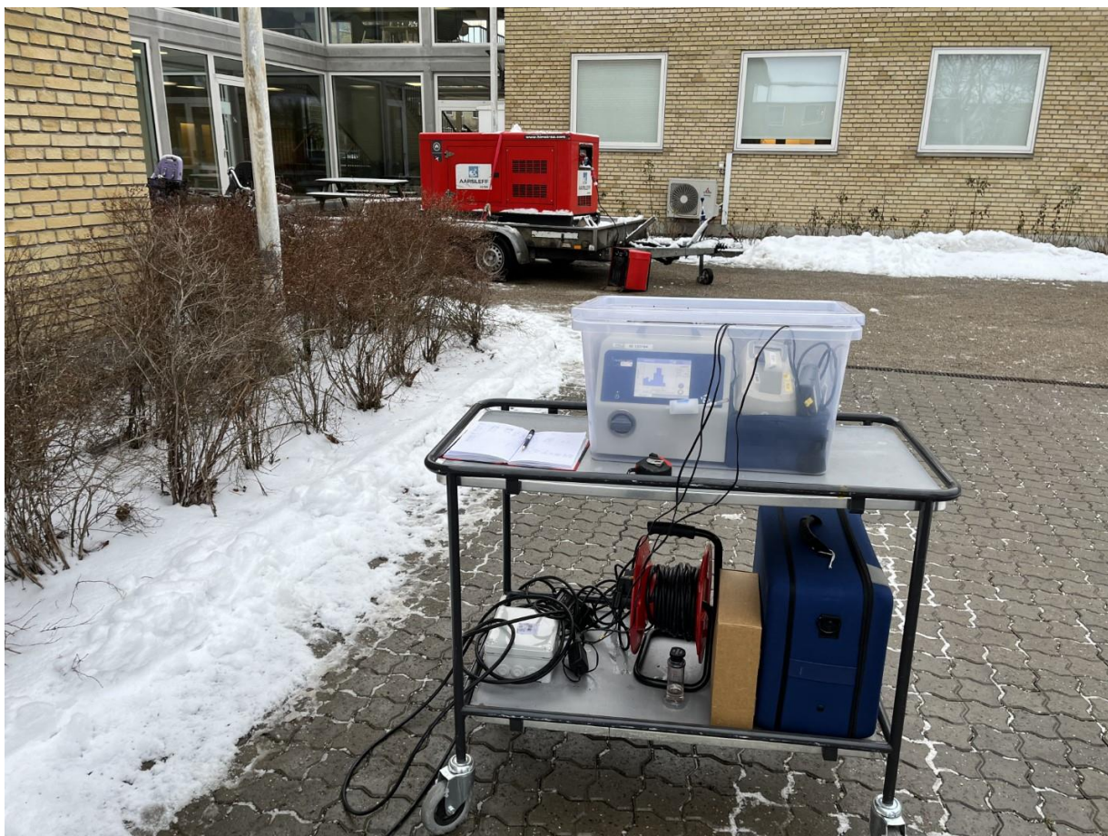
Figure 8. Measurement position 4, 700-800 cm from the diesel generator.
